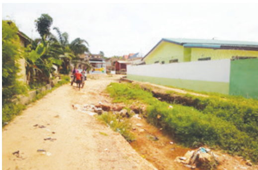
Fig 2.8 Typical road supposed to be the shortest route to flood prone area for emergency responders at AnteAku, near Santa Maria
