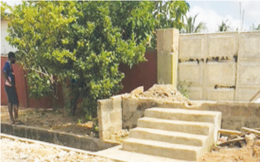
Fig 2.4 Efforts to mitigate floods include continuously heightening barriers at entrance points.
